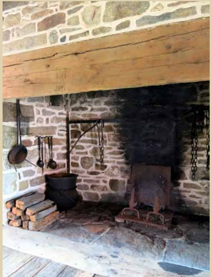
Colonial-era cooks stepped among the coals to prepare meals in hearths such as this 14-foot-wide example in the home of Ken Muth of Bucks County, Pennsylvania. This one features an iron crane, an innovation replacing the dangerous lug poles of the earlier period.
