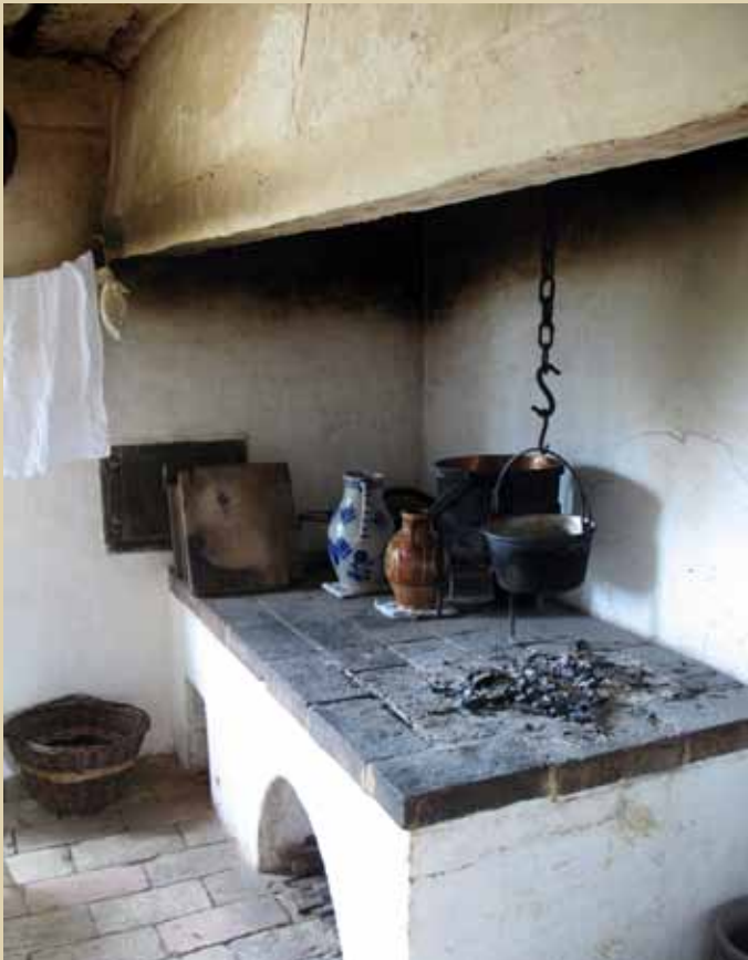
During the 1700s, German and Dutch colonists in America brought the concept of the raised hearth from their homelands. Heated from underneath the stovetop, these hearths relied on overhead chimneys. They reduced the amount of bending the cook had to do, as well as improved protection of the cook from the fire. (Frontier Culture Museum in Staunton, Virginia)
