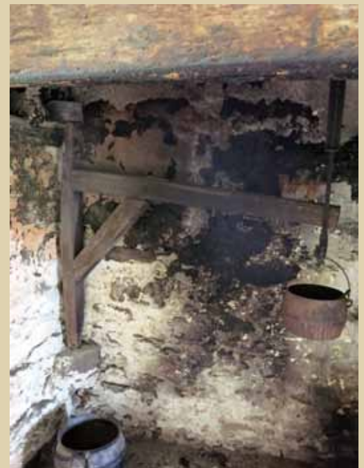
This early walk-in hearth has an original, rare wooden crane for holding pots over hot coals. Cranes replaced the more dangerous lug poles during the 1700s, though most cranes were made of iron. This hearth is in the Pennsylvania home of Bernie Bogotnik.
