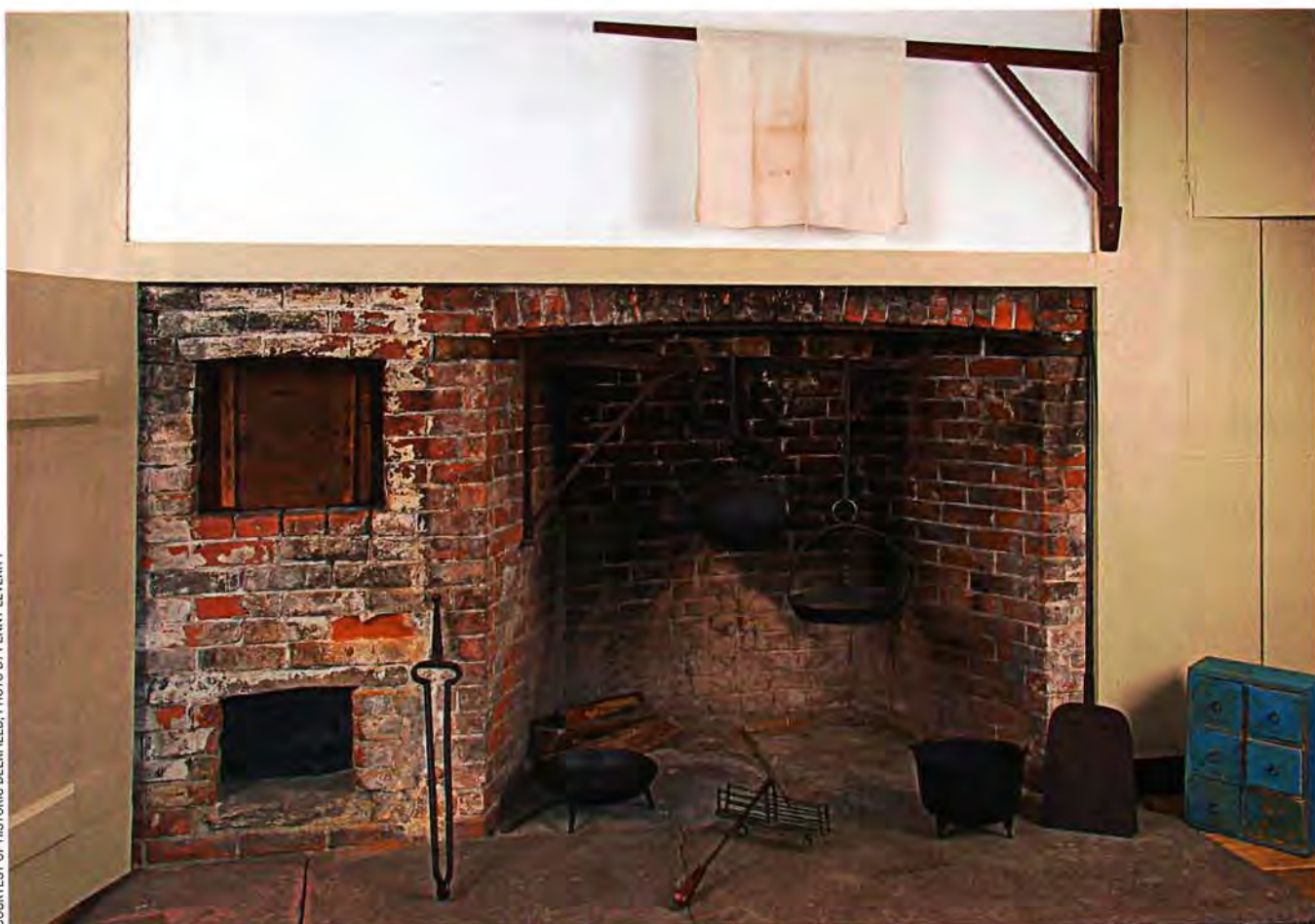
The hearth in the north kitchen of the Sheldon House at Historic Deerfield in Massachusetts is an excellent example of a late-18th-Century transitional fireplace. Still tall and wide like typical cooking hearths in the mid-1700s, it also has angled sides resembling a late-1700s Rumford fireplace. An oven built to the left of the hearth is heated from the firebox below it. The Sheldon House dates from 1754, but an 1802 addition contains this kitchen.
